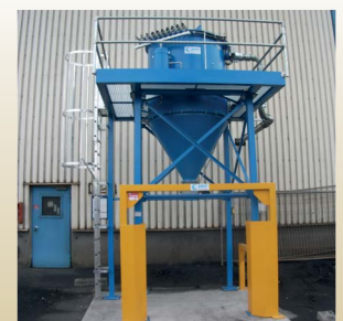
Filter pre-separator with constructive explosion control and decompression
